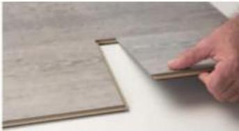
2. Slide the plank until it reaches the short side of the next plank and drop gently.
