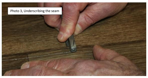
3. Cut the seam using a utility knife (straight or hook blade). Cut the seam by following the scribe mark. Your fall off should be to your right if you are right handed and to your left if you are left handed (see Photo 4).
